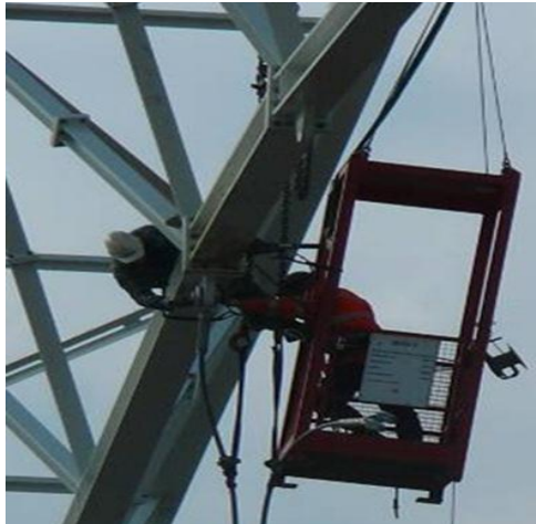
3 Team work for complex steel construction assembly
