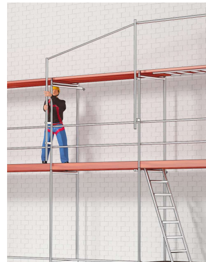
Figure 3: Temporary guardrails assembling
