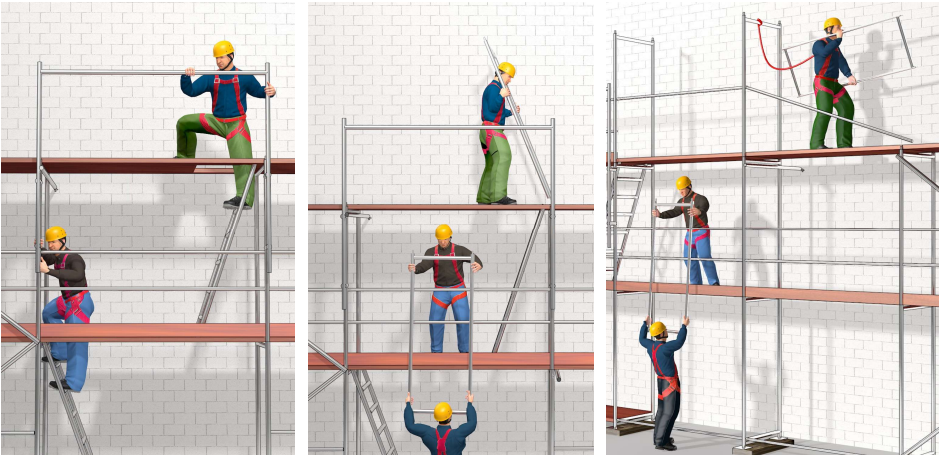
Figure 5 to 7: Scaffolding erection with PPE and temporary guardrails
