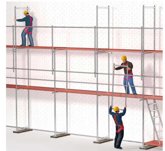
Figure 4: safe Scaffolding work with temporary guardrails
