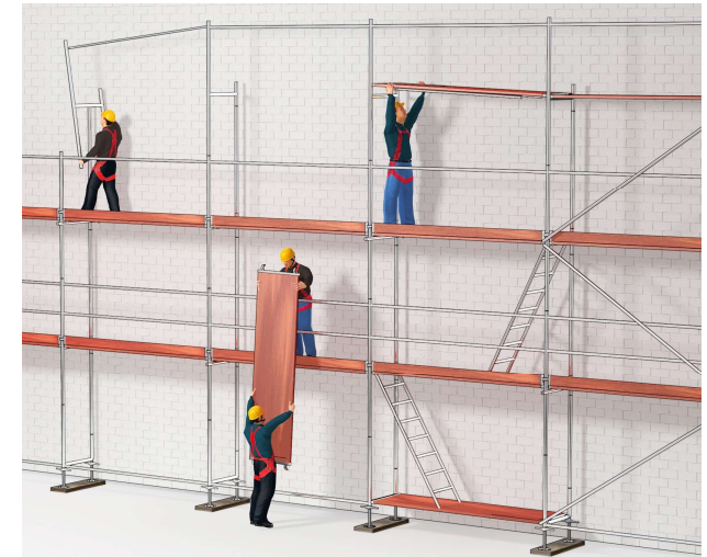
Figure 2: frame with build-in guard rail while erecting scaffolding
