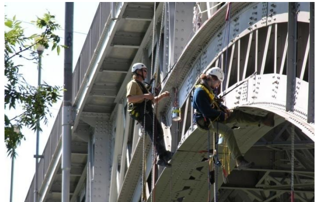
1. Rope access always requires redundant safety measures.
